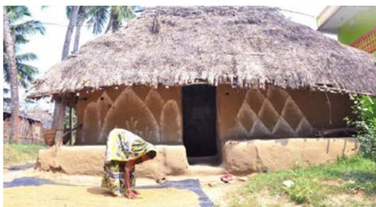
**Fig. 3.** A typical structure of house built by farmers and other people in rural areas where they stay as well as store their harvested agricultural products. Roof is made up of rice straw and the walls are made up of clay. (Photo source: <https://www.mycitylinks.in/why-this-village-in-odisha-has-no-doors>).
